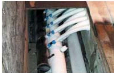
Figure 12. Plastic rink piping connections to the distribution and the collection mains (thermally insulated).
